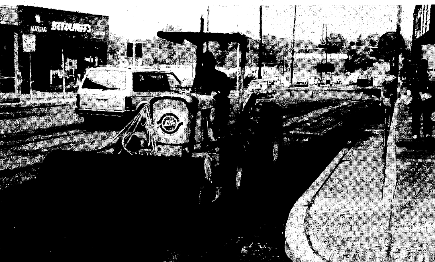
A ROTATING METAL BRUSH is used to mill off old asphalt on Main St. as the state is preparing to put down a new blacktop surface from Chelsea Community Hospital on the south to Sibley Rd. on the north. The work has caused traffic back-ups in both directions. The village is scheduled to begin the same kind of work on both E. and W. Middle Sts. this week.
