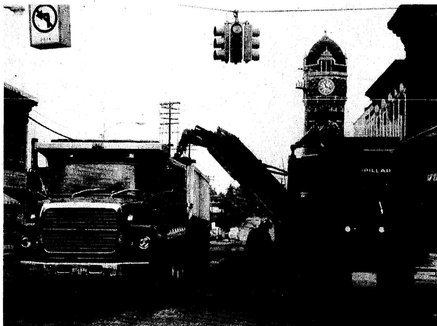
ROAD WORK on M-52 continued through the center of town last week and this week as state workers milled asphalt down to the road's concrete base. The village looked like a ghost town as no parking was permitted on the streets and often no traffic was allowed through town. The project is supposed to be finished by Nov. 15.
